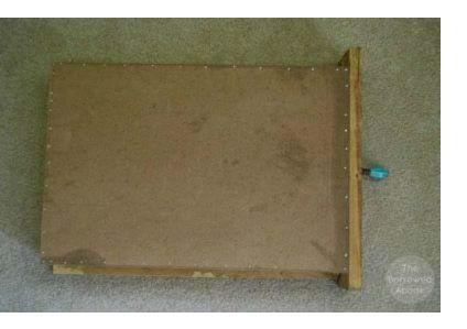
Once the drawer frames are dry, attach the MDF bottom using more wood glue and small nails.
